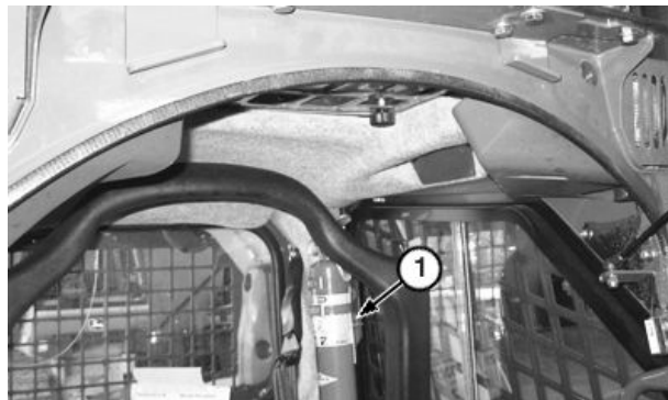
Fire Extinguisher Location
